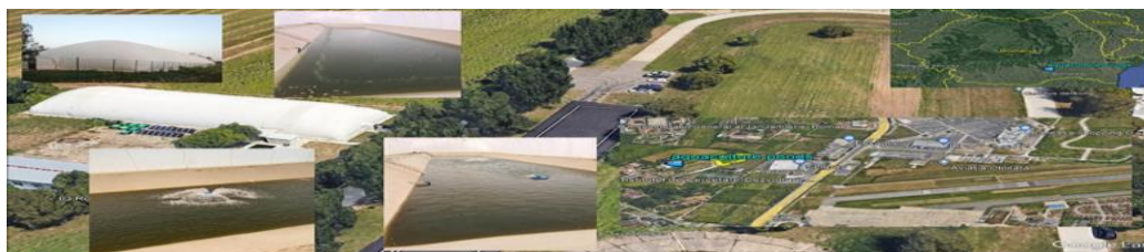
Fig. 1 - Basin no. 1 (ICP1), covered pool and the location with details, the inside of the pool with water quality maintenance devices. The coordinates are 44° 30' 9.51" N, 26° 4' 21.94" E
